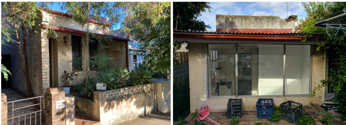
Figure 3: Site viewed from Victoria Street and from within the rear yard
