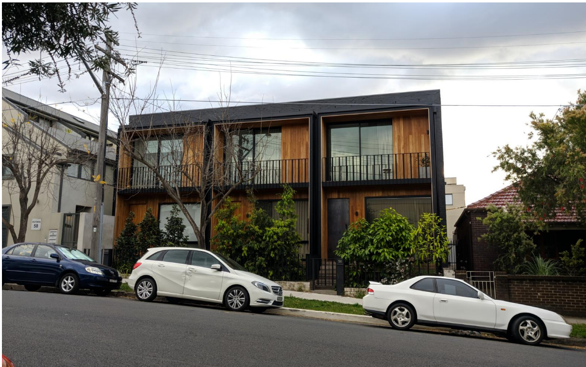
Figure 5: 56, 56A and 56B Victoria Street located to the south of the site, consisting of 3 x attached terrace dwellings within an adaptively reused former warehouse building (2019 photograph taken by Council officer)
